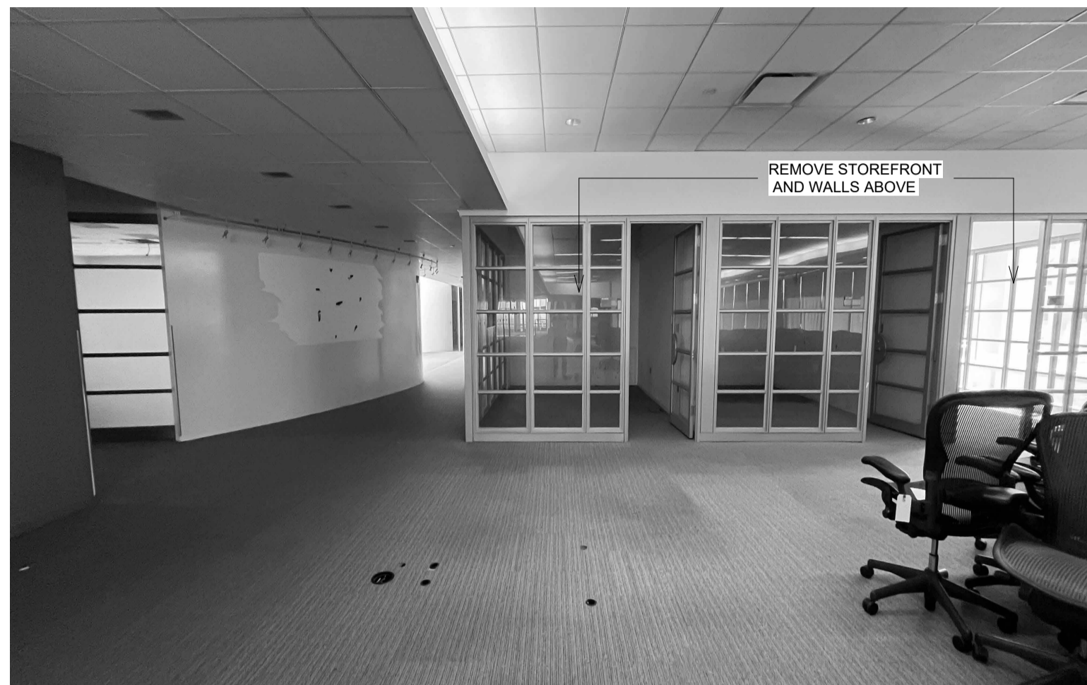
EXISTING OFFICES, FACING EAST
