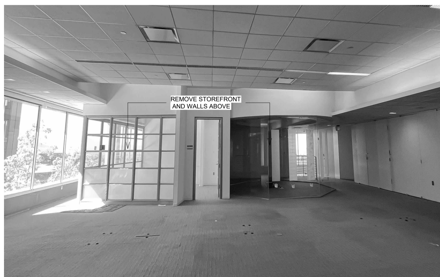
EXISTING OFFICES, FACING WEST
