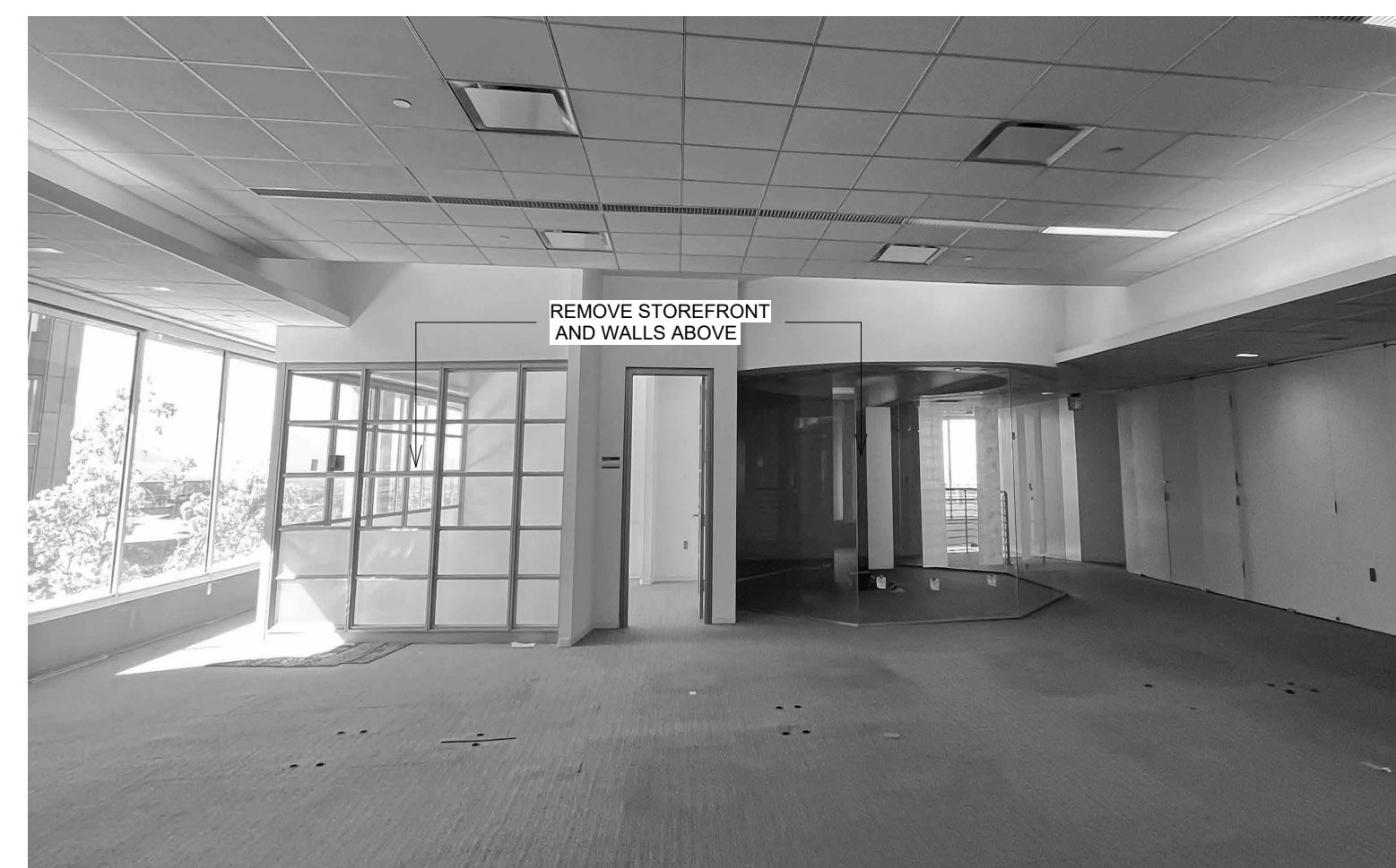
EXISTING OFFICES, FACING WEST
