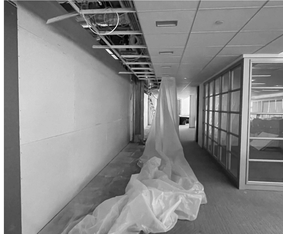
ENTRANCE HALLWAY, FACING EAST
