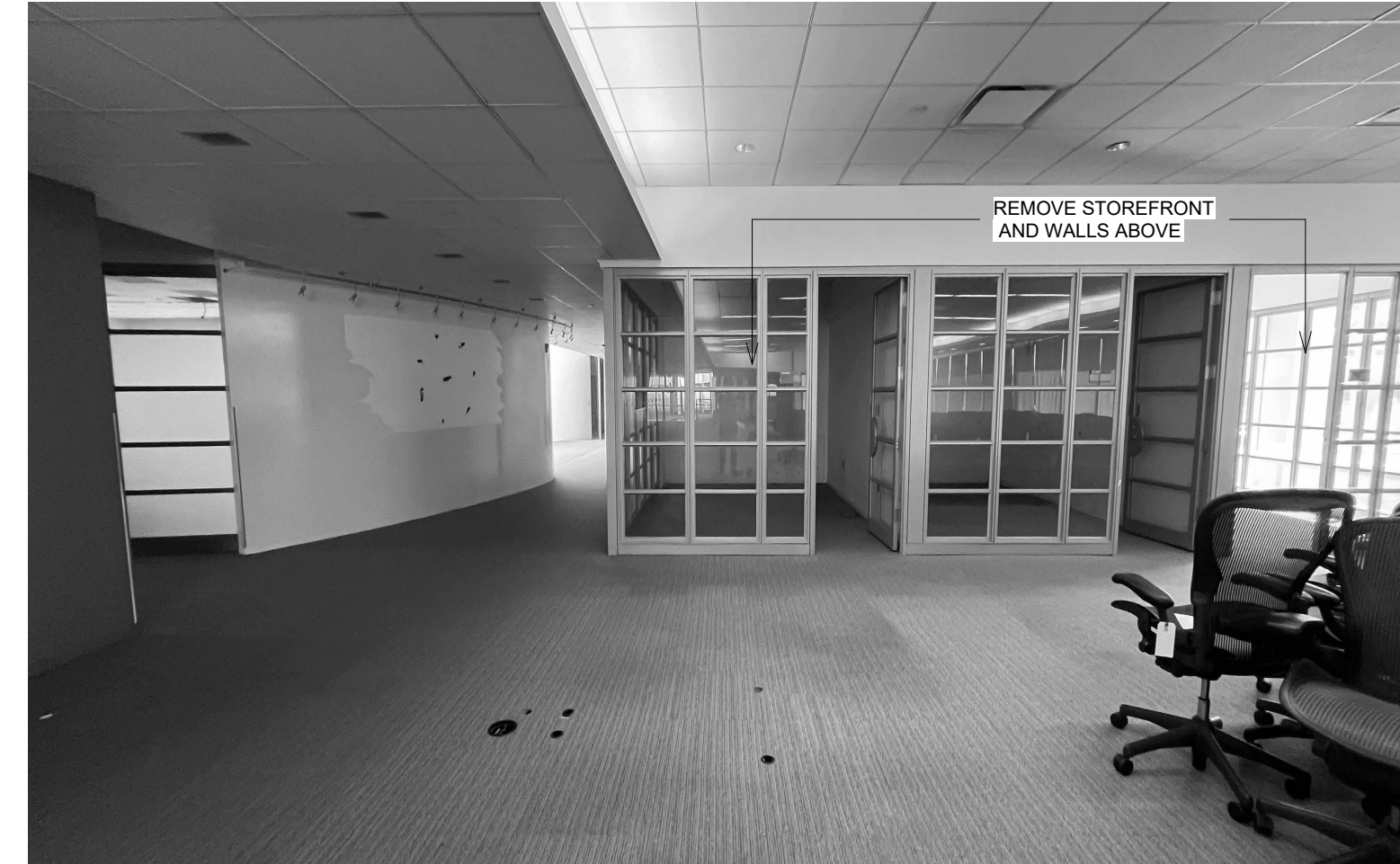
EXISTING OFFICES, FACING EAST
