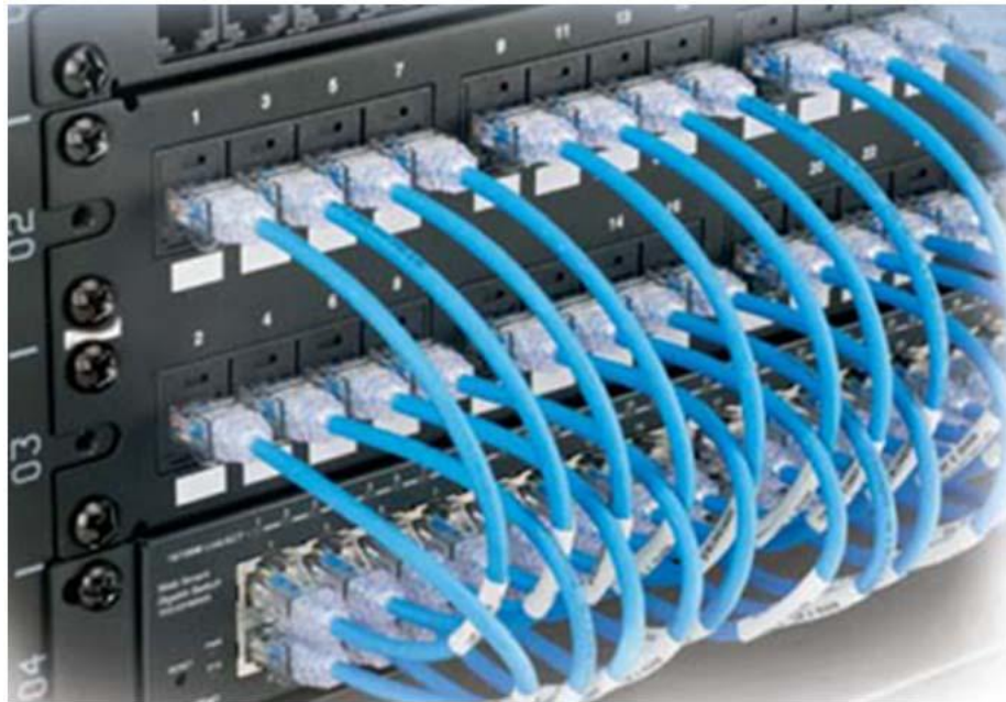
Example of one-to-one switch patching
